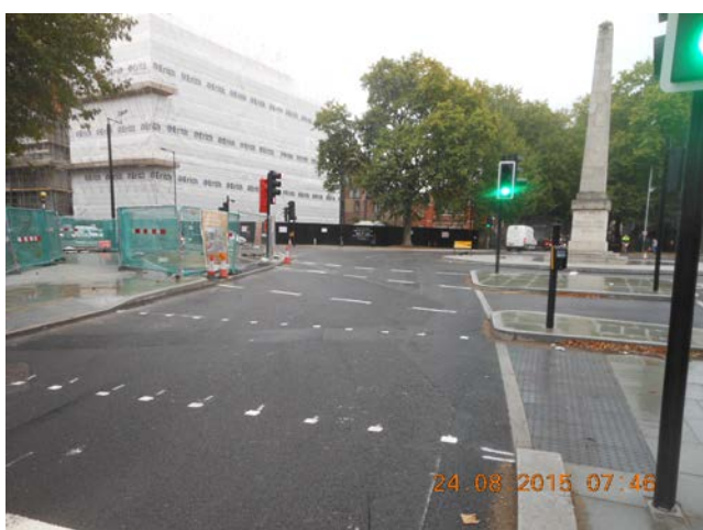
Works in progress at St George's Circus
