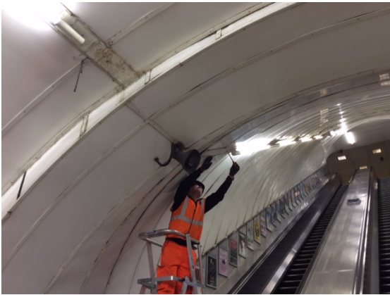
Survey works at Liverpool Street
