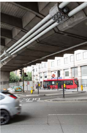
Expansion joint installation at Hammersmith flyover
