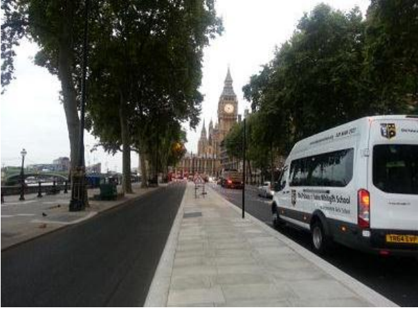
Newly opened section of cycle track between Derby Gate and Horse Guards Avenue
