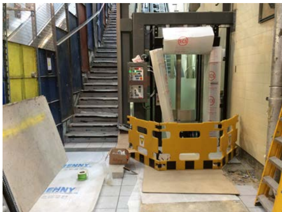
Lift works in progress at Greenford station
