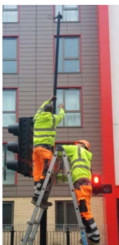
Installation of Split Cycle Offset Optimisation Technique (SCOOT) technology
