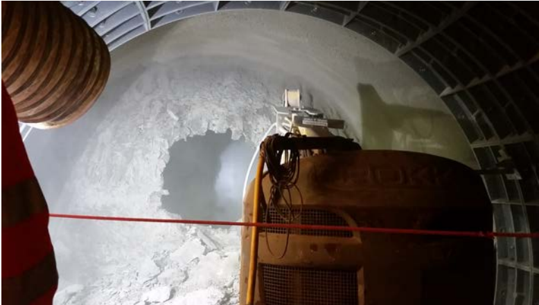
Tunnelling breakthrough at Bond Street station upgrade
