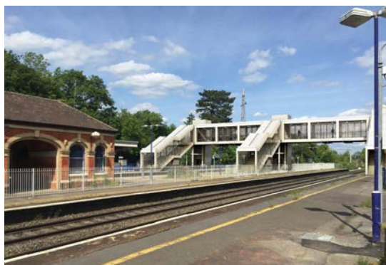
Standard new footbridge to be provided at Manor Park and Seven Kings, with full height glazing requested by users to increase safety
