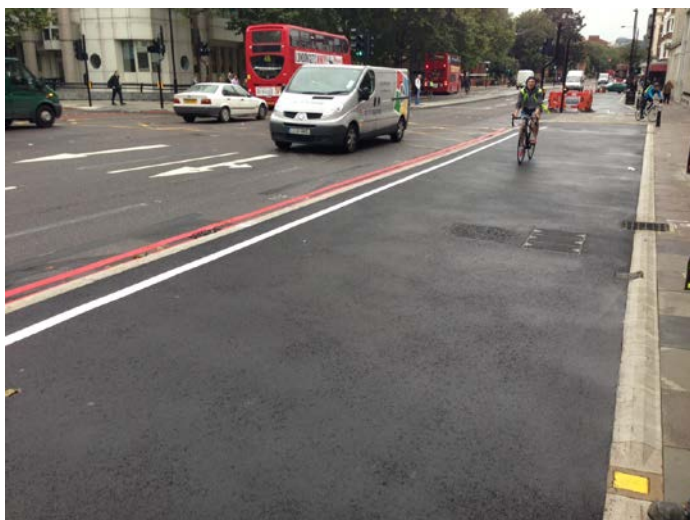
New cycle track on A202 Vauxhall Bridge Road (Cycle Superhighways Route 5 Inner)
