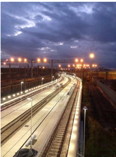
New sidings at Wembley
