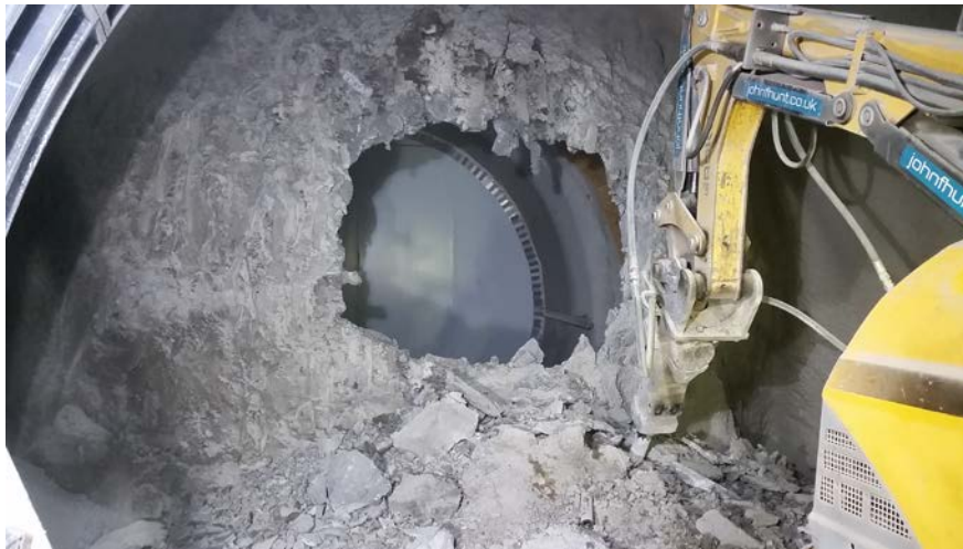
Tunnelling breakthrough at Bond Street station upgrade
