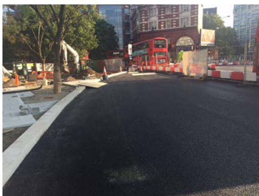
New widened carriageway at London Road junction
